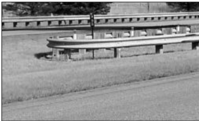
Above - "W-beam" bullnose guardrail has been used in Nebraska for many years.
