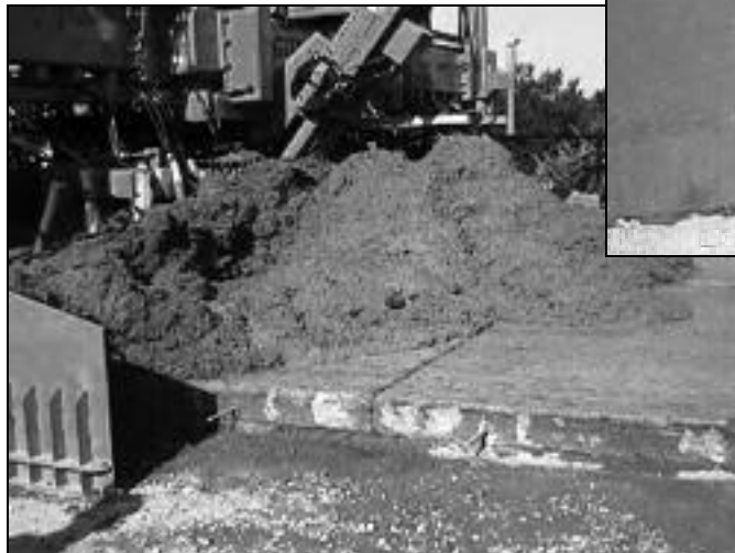
Left - 3M fiber-infused concrete in front of paver is prepared for placement.
