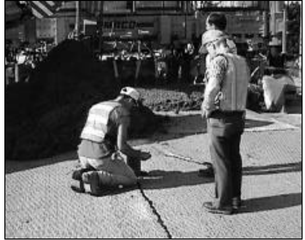
NDOR workers obtain a core sample for testing.
