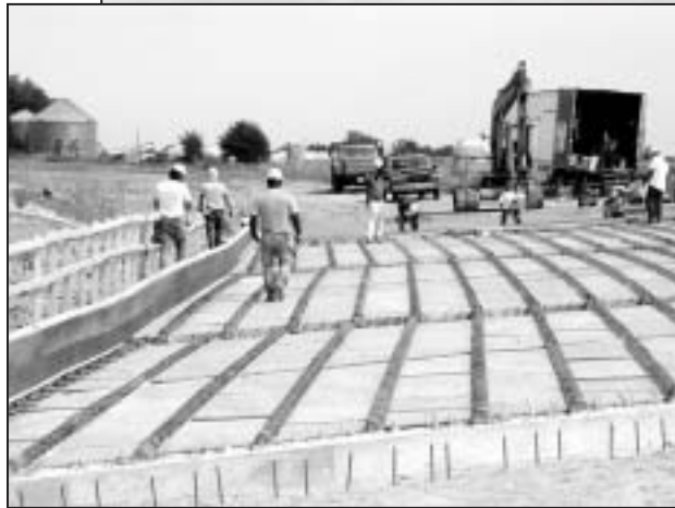
Above - Recently completed segment of Highway 81 near Geneva. Left - Workers are preparing a bridge deck on Highway 81 near Geneva.
