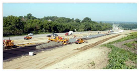
Payment operations are underway on West Dodge Road (Hwy 6) just east of the Elkhorn River. Cement trucks (top) line up to deliver their loads and a slipform payer (bottom) forms concrete for the new roadway surface.
