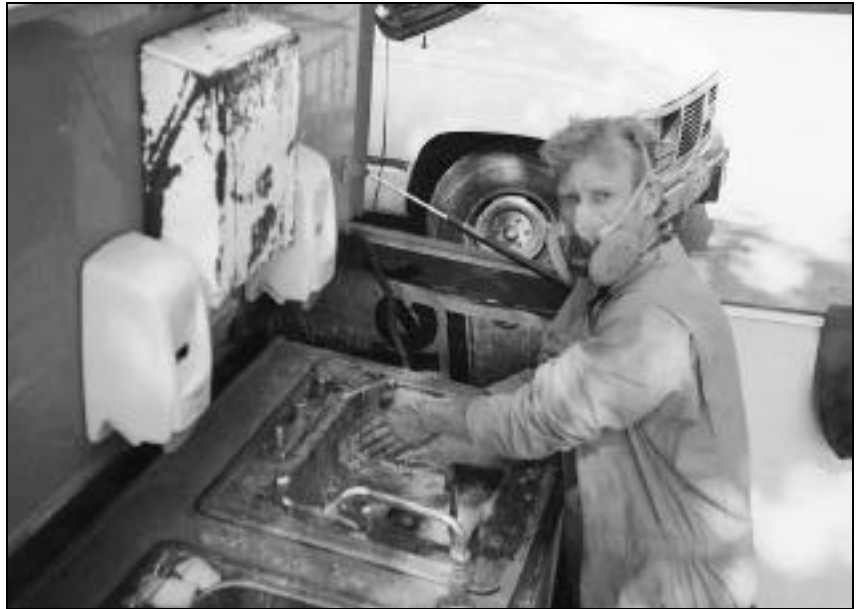
Protective clothing and breathing apparatus are required for sandblasting and painting operations.
