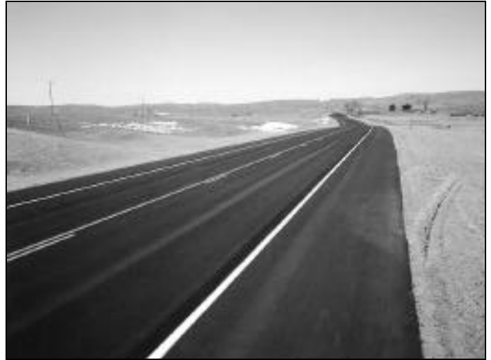
This completed section of Highway 83 is located on the north end of the project.
