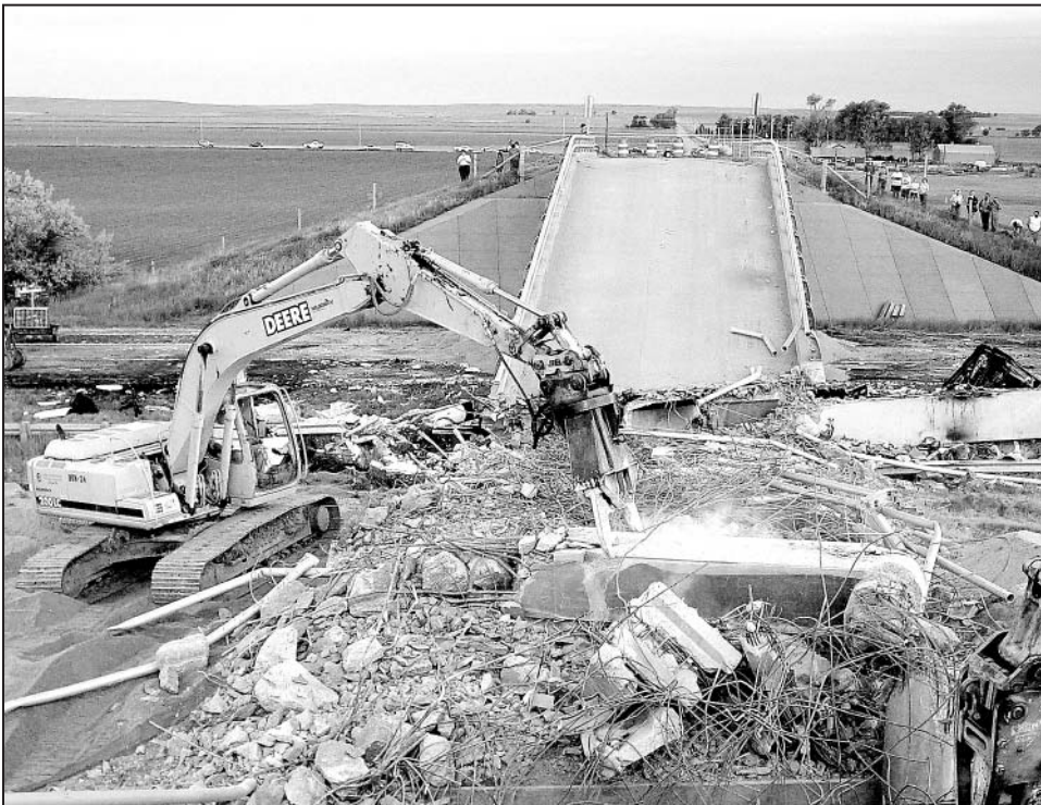
Working on a cushion of sand, the heavy equipment began the job of tearing apart the overpass so it could be hauled away.
