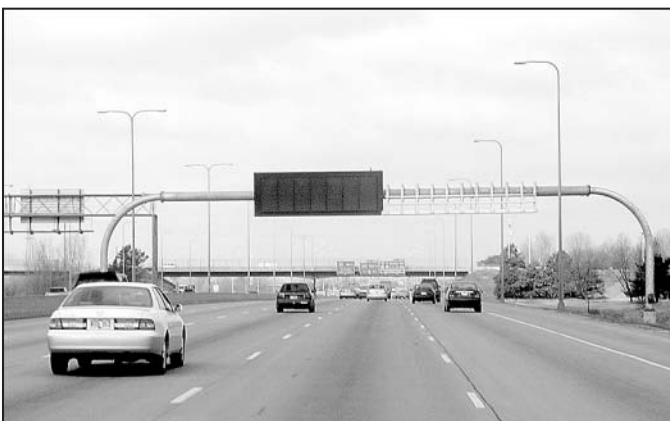
Looking westbound, this dynamic message sign is located on Interstate 80 at approximately 94th Street in Omaha.
