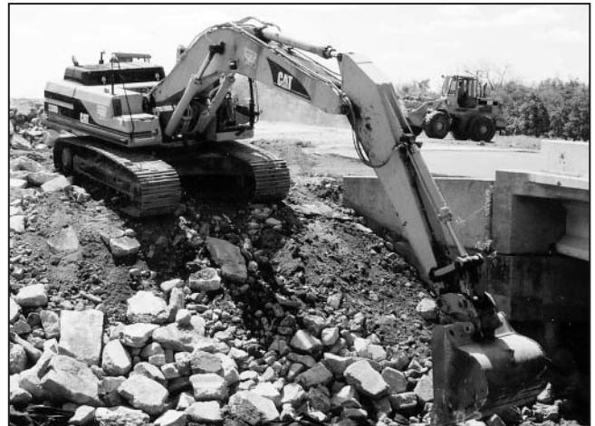
Riprap is being utilized to stabilize the banks to prevent erosion.
