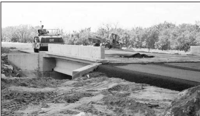
Asphalt is being applied to the subgrade to smooth the approaches to the bridges.
