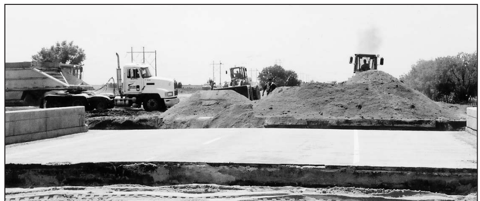
Heavy machinery puts in the subgrade on the approaches to match the bridge slabs. Top left - Lines formed as traffic was diverted at the Brule interchange.
