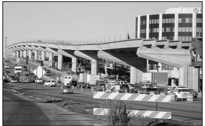
Westbound Expressway Bridge taking shape.
