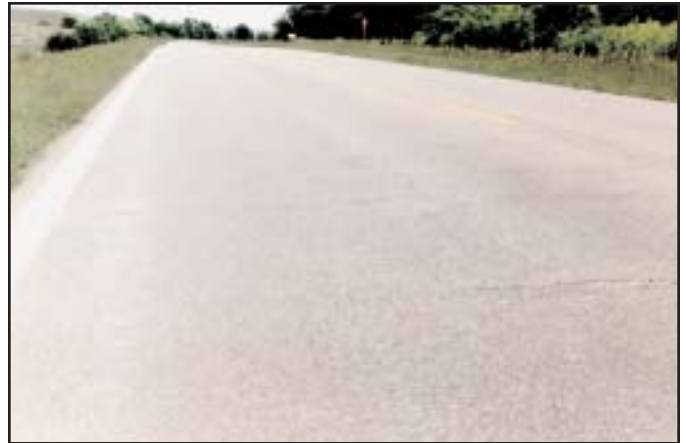
Low - Slight waves, sags, humps, corrugations or wash boarding of the pavement.
