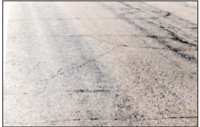
Low - Hairline cracks, essentially transverse but may connect to longitudinal; spacing of 50 to 100 feet.
