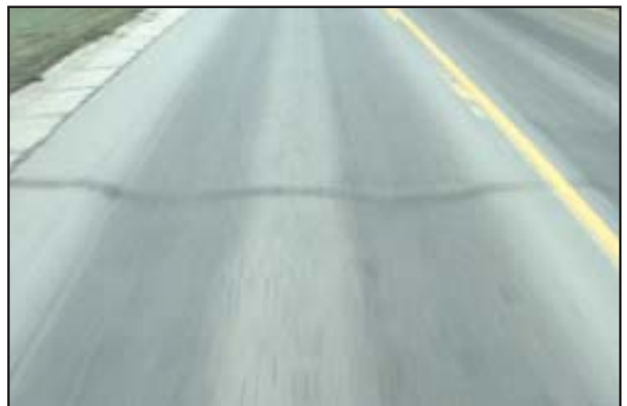
High - Wheel path depressions greater than \frac{1}{2} -inch.
