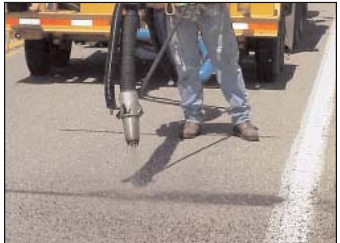
Figure 5.15 Spray Injection (AMZ)
