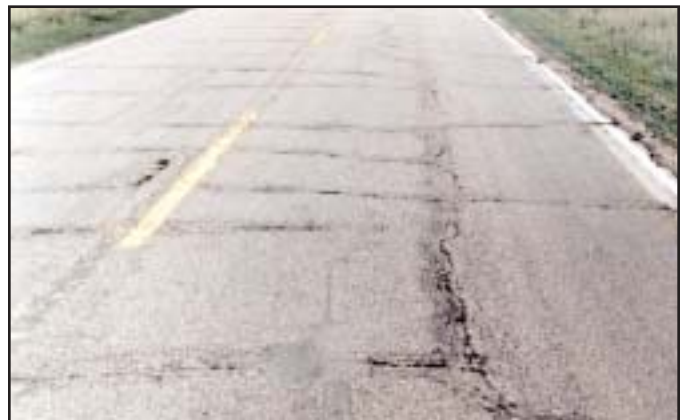
High - Cracks greater than 1/8-inch wide that are random or have a block pattern, similar to a turtle shell.
