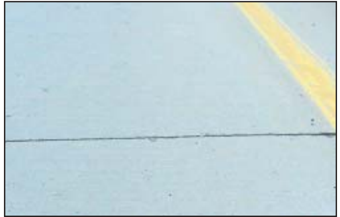
Low - Less than \frac{1}{8} -inch vertical displacement between adjacent panels.
