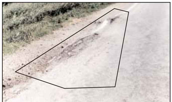
High - Shoving and major changes in pavement profile that require vehicles to slow from normal speeds.
