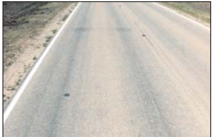
Moderate - Wheel path depressions of \frac{1}{4} - to \frac{1}{2} -inch.
