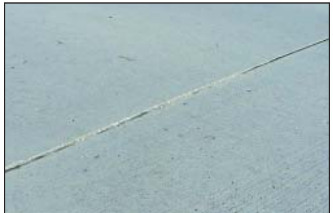
Moderate - Displacement of \frac{1}{8} - to \frac{1}{4} -inch between adjacent panels.
