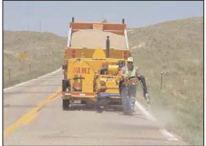
Figure 5.14 Spray Injection (AMZ)
