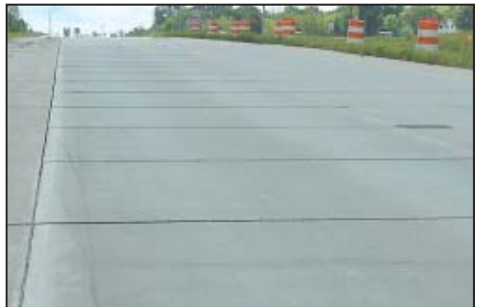
High - Displacement greater than \frac{1}{4} -inch between adjacent panels.
