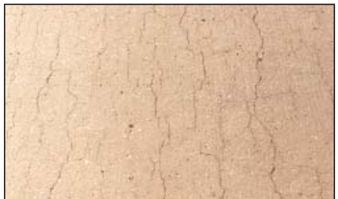
High - Occasional to extensive interconnecting cracks \frac{1}{8} -inch wide or greater. Spacing between cracks is usually only a few inches.
