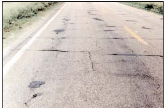
Moderate - Cracks range from hairline to 1/8-inch wide and may be slightly spalled.
