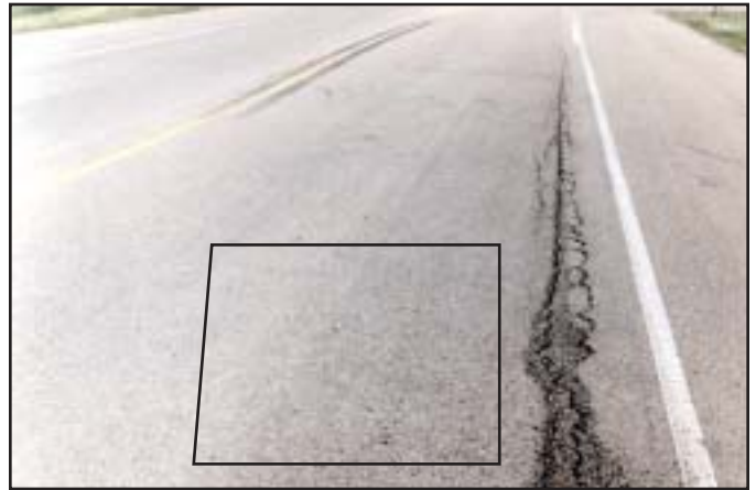
Low - Minimal loss of aggregate or binder.
