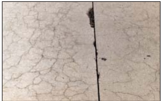
Moderate - Frequent hairline to \frac{1}{8} -inch cracks radiating from the joint forming a web like pattern.
