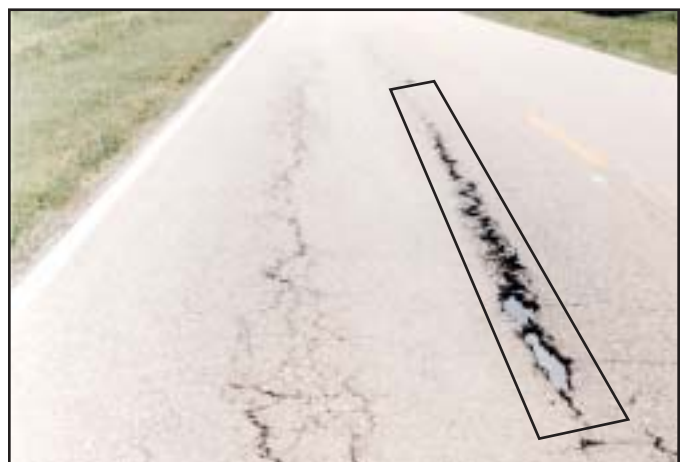
High - Single cracks are wider than 1/8-inch.
