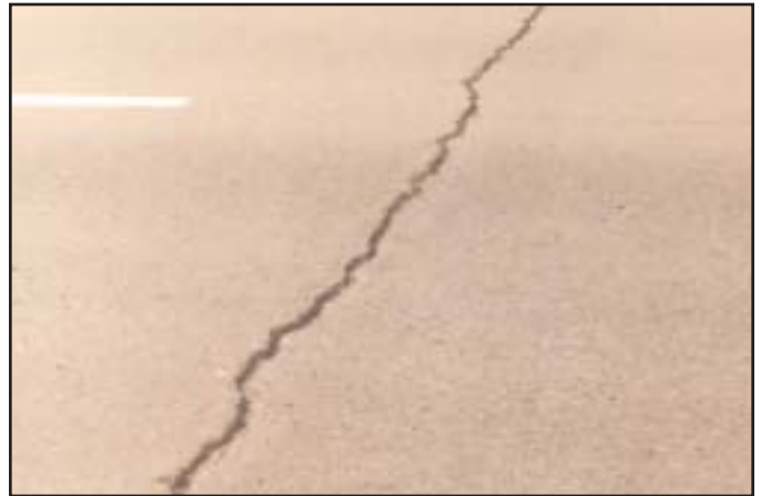
High - Transverse cracks greater than \frac{1}{4} -inch wide extending the full width of panel.
