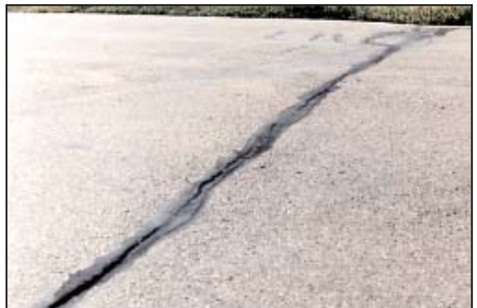
Moderate - Similar to low except distortions can be felt while riding in a vehicle.
