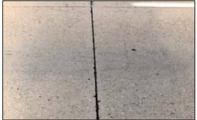
Low - A few hairline cracks from the joint and/or discoloration at the joint.
