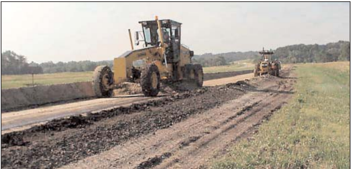
Figure 5.16 Machine Patching
