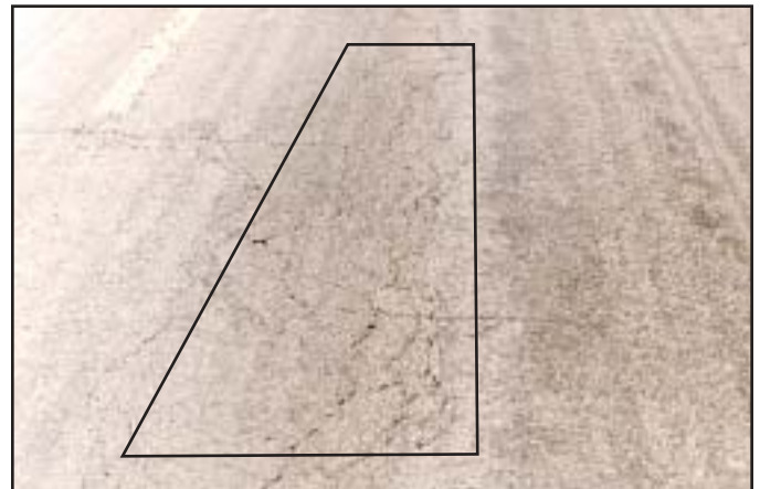
Moderate - Longitudinal cracks in wheel paths forming an alligator pattern; cracks may be lightly spalled and about \frac{1}{8} - to \frac{1}{4} -inch wide.
