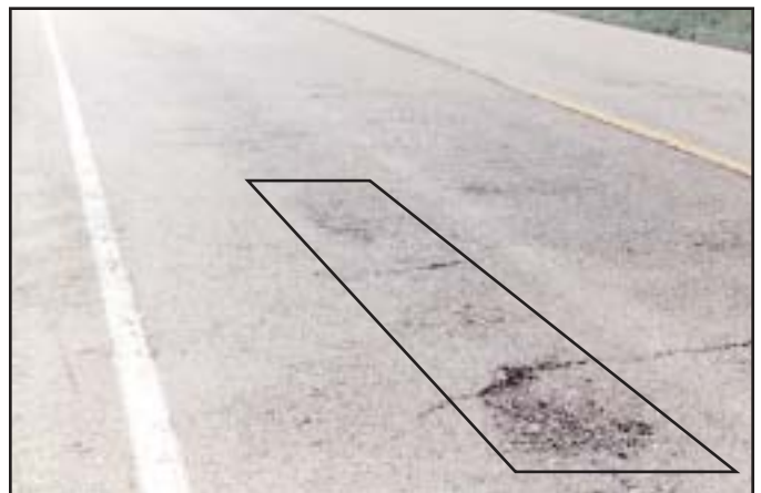
High - Sections greater than one square foot may be pitted, stripped or eroded away.
