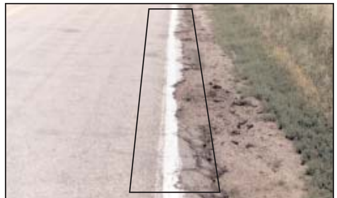
High - Cracks greater than \frac{1}{4} -inch; may have loose or missing pieces or potholes or alligator cracking.
