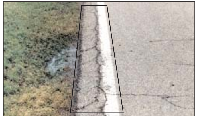
Moderate - Cracks \frac{1}{8} - to \frac{1}{4} -inch located 1 to 2 feet from the edge of the road; may have an alligator pattern.
