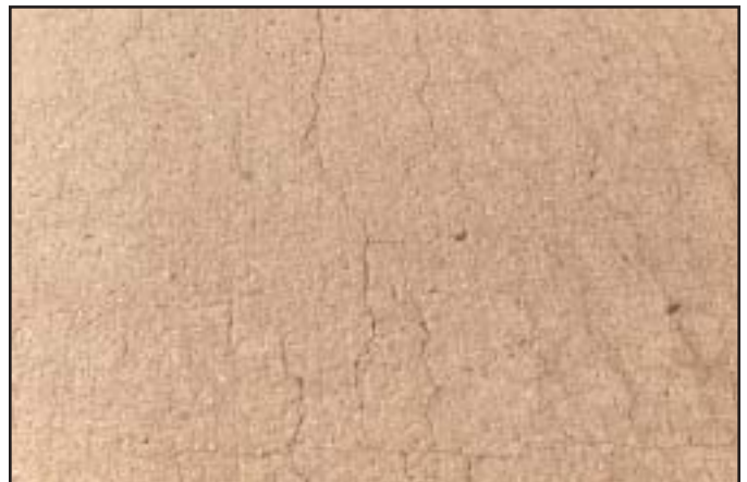
Moderate - Interconnected cracks between \frac{1}{16} - to \frac{1}{8} -inch wide throughout the panel.
