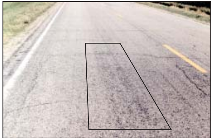
Moderate - Some aggregate loss; small areas may be stripped away.
