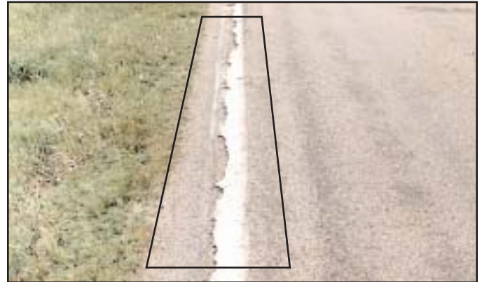
Low - Hairline cracks just beginning to show; random with no pattern; may be up to \frac{1}{8} -inch wide.
