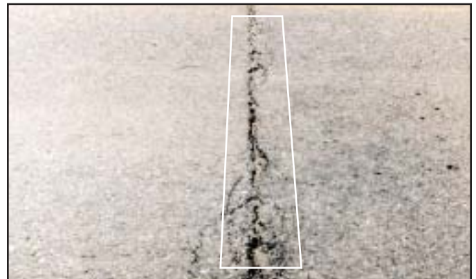
High - Cracks \frac{1}{2} - to 2-inch wide; larger cracks often are spalled and/or have noticeable distortions near them. Cracks greater than 2 inches wide and causing extremely rough ride are rated "X".
