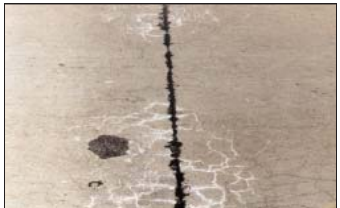
High - Cracks \frac{1}{8} -inch or larger forming multiple patterns and often having a white appearance.
