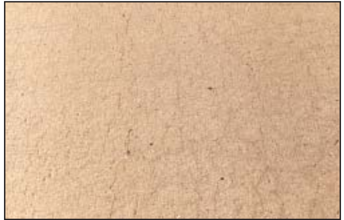
Low - Negligible or occasional interconnecting \frac{1}{16} -inch wide or less cracks.
