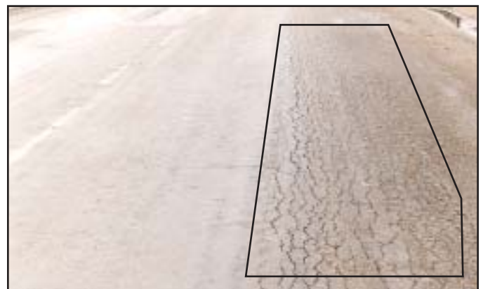
High - Pieces appear loose with severely spalled edges; cracks are \frac{1}{4} -inch or greater and pumped fines may appear on the surface.
