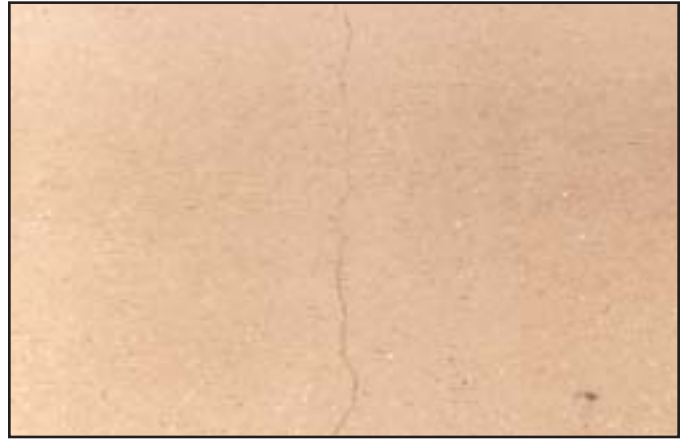
Low - Hairline to \frac{1}{4} -inch wide cracks extending the full width of a panel.
