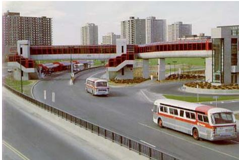
A busway is a roadway for the exclusive use of transit buses. The typical configuration is two lanes (one for each direction), with pull-out lanes at stations so express buses can pass locals, and ramps as required to/from other highways and streets.
