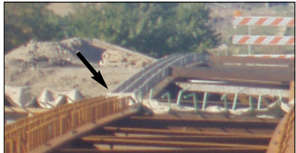
Box girder design which was used on Highway 2 bridge at Grand Island. Note the discontinuity of the girders at the pier, showing two distinct arches. This is the first high performance steel 100 (HPS100) bridge built in the United States.
